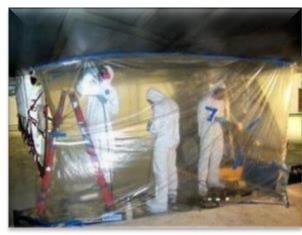
Airmen sanding degraded paint coatings within an enclosure to contain hazardous material generated during de-painting.
