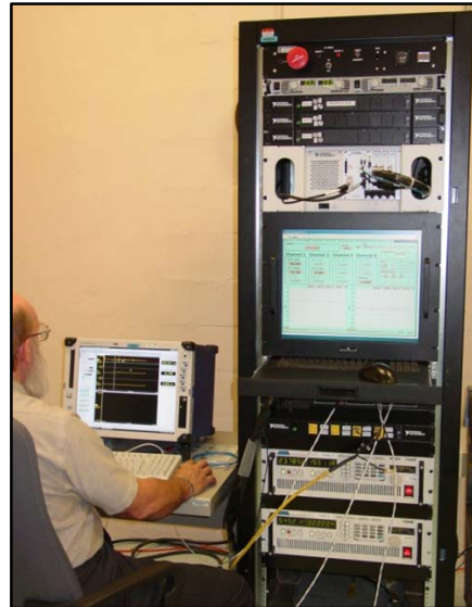
Programmable Testers and High-Speed Data Acquisition
