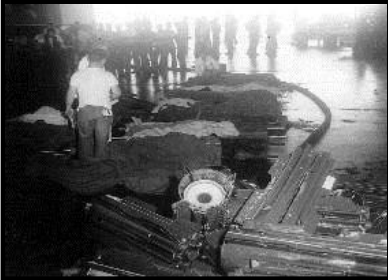
Hole in deck
