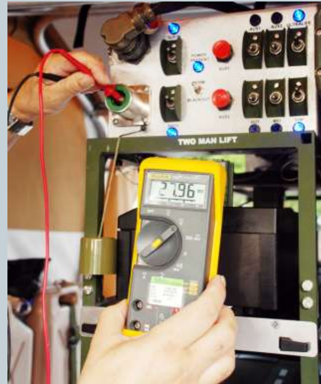
Power Distribution & Protection
