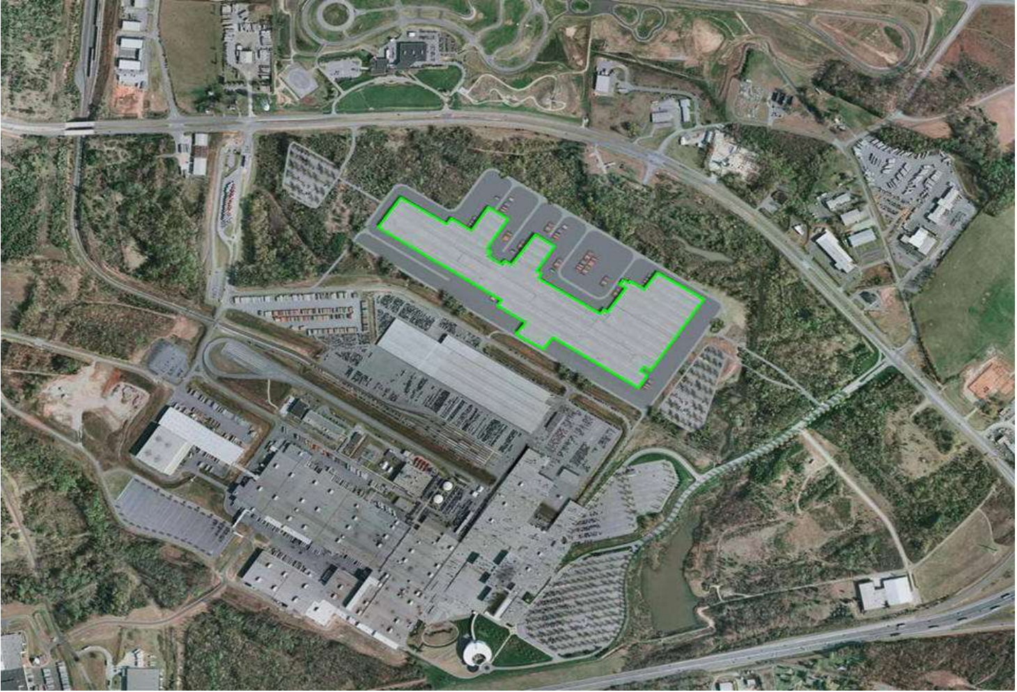
BMW X5 and X3 Production Facility, Greer, SC
