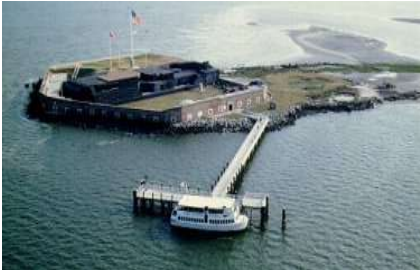
Planned Site for Ft. Sumter Renewable Energy Project, Fall 2010
