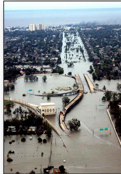
Hurricane Katrina Flooding
