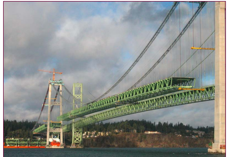
Tacoma Narrows Bridge 2006
