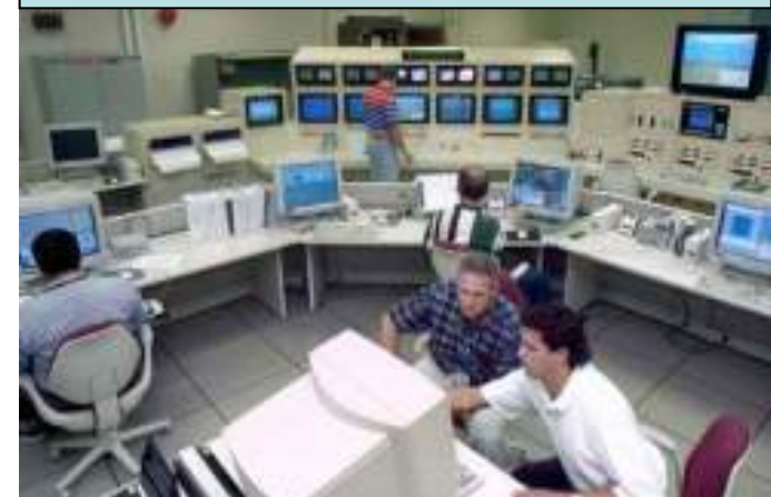
Simulation Computers and Control Room
