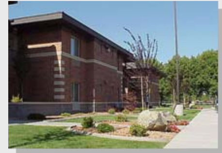
The Guest House at PNNL
