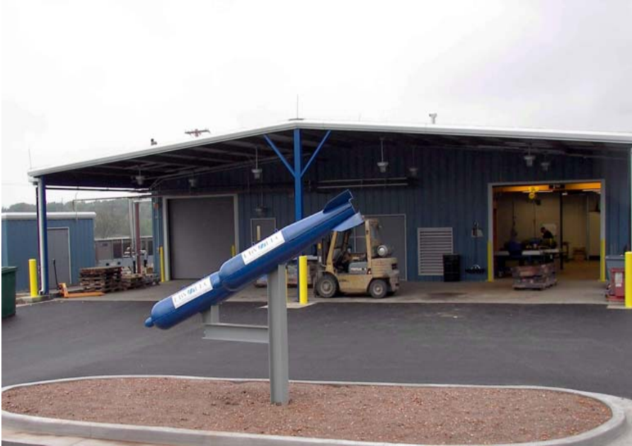
New CBU Building
