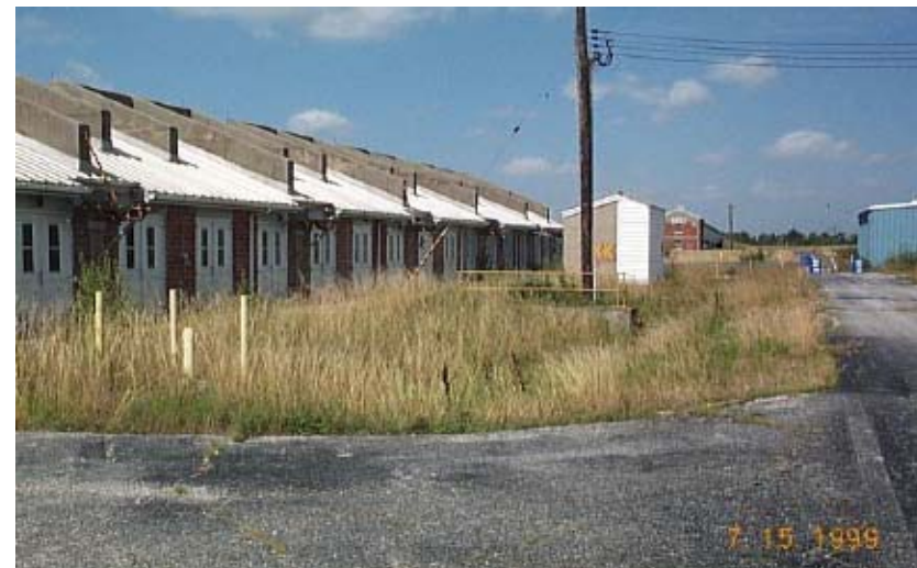
Building Remediation or Demolition Kansas AAP
