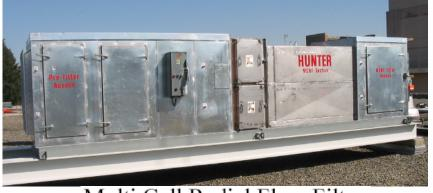
Multi Cell Radial Flow Filter Housing
