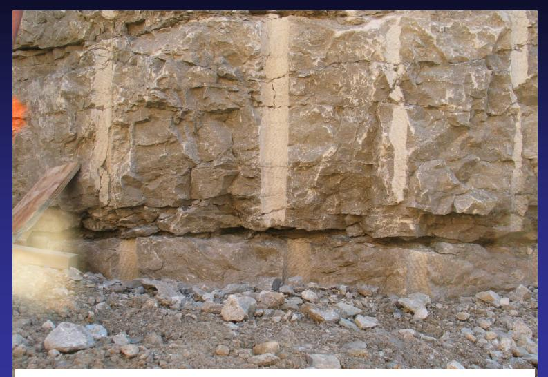
Offset boreholes observed in north face of north culvert
