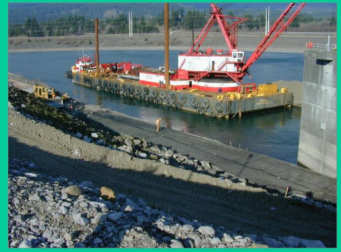
To provide separation, improve foundation bearing, and drainage for the Transportation Channel slab, a compacted bedding gravel layer on a Geotextile Fabric was constructed. The Transportation Channel slab was then formed and placed on the bedding.
