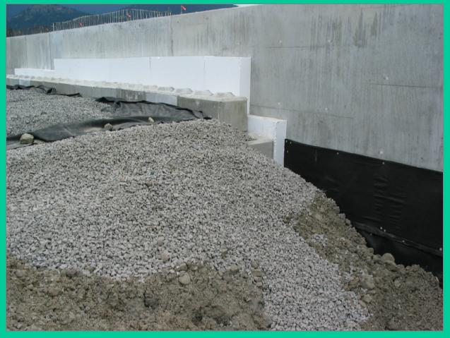
Contractor VE Proposal - use a MSE embankment to backfill an open cut was accepted for the upstream portion of the Channel wall. Originally a soil nail wall and top-down excavation had been planned - but the elected open cut remained stable.
