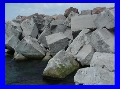
Used initially in "Laid Up" structures Later used in rubble mound and as capstone
