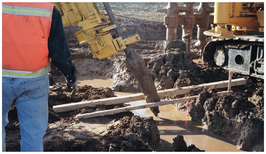
Sampler plugged with soil from unimproved zone
