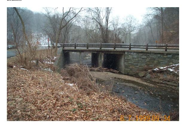
Photo below shows the downstream face of the Broad Branch Road bridge over Broad Branch. There is a concrete shelf across the channel immediately downstream of this bridge. The drop off is 3-feet in height.
