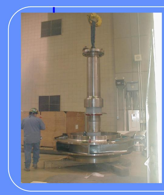
Pump Propeller is ready to be dropped from +45' to the pumphouse at -297' below.
