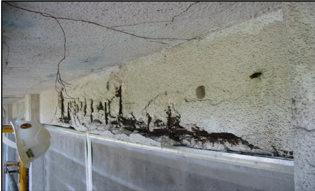
Corrosion of rebar and spalled concrete in the west side beam
