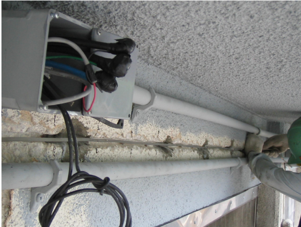
Discrete anode system being installed in the west beam
