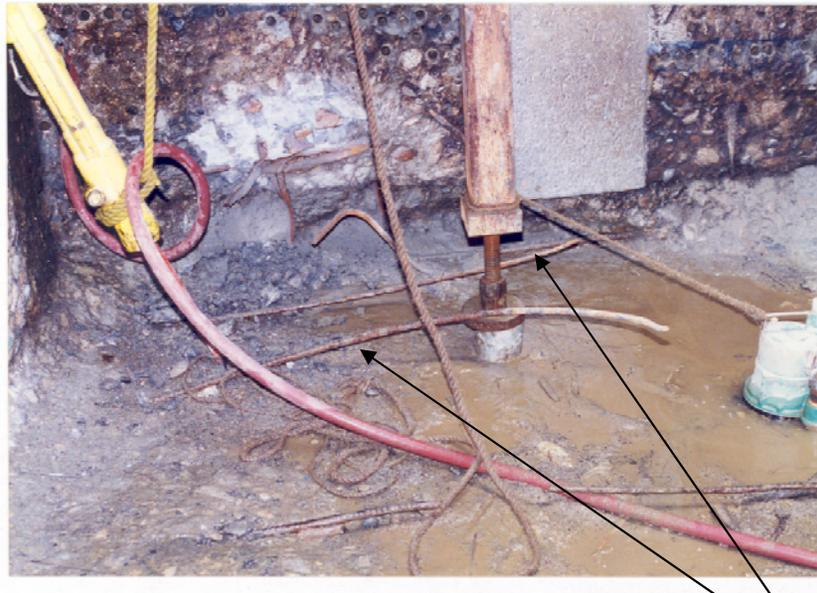
Note close-up of damage of exposed and worn rebar in scour hole prior to repairs
