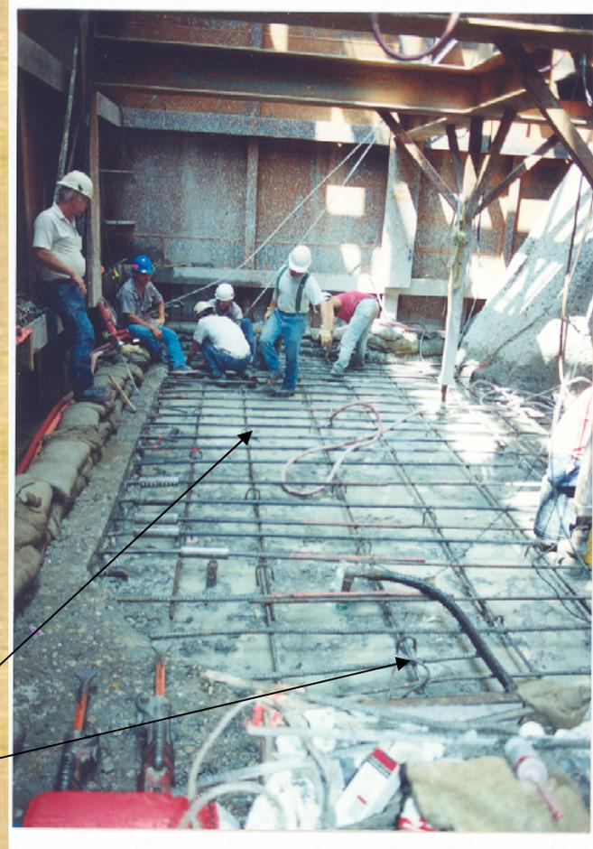
Limits of scour hole and repair of missing and damaged rebar throughout entire area around nose pier
