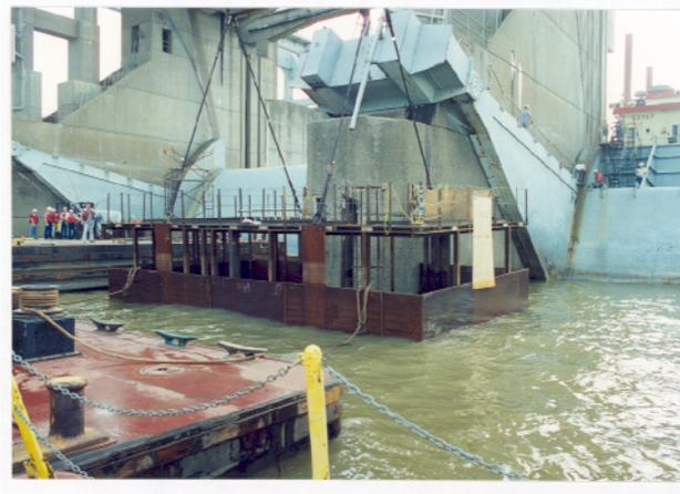
Temporary dewatering box built by LRS to make limited scour repairs around piers at the Markland Project.
