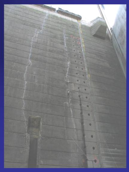
**John Day Navigation Lock Concrete Rehabilitation**  Monolith Joint Isolation/Sealing •Concrete Repair Monolith 6 Concrete Lift Sealing •Crack Sealing/Repair Backfill Drain Rerouting
