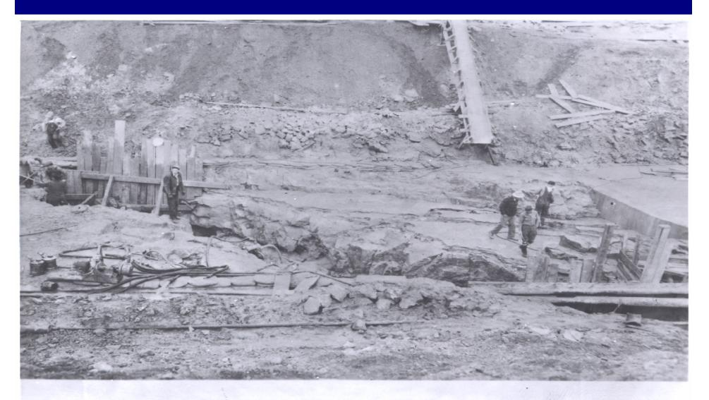
Looking NW from 35' U.S. of station 40 / 15: Open joint in cut-off trench foundation.
