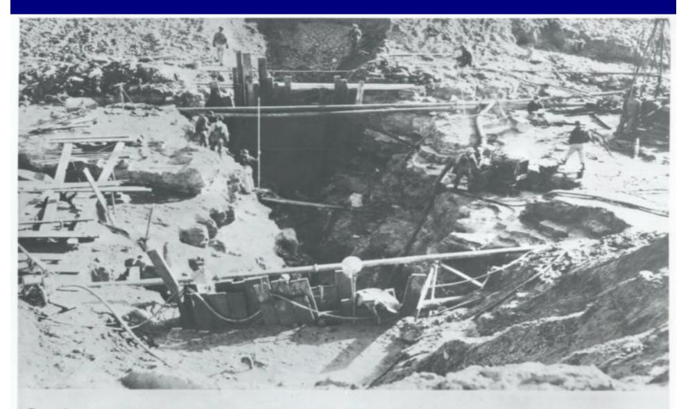
Looking S from 175' US of station 39 / 20: Open joint in cut-off trench foundation.
