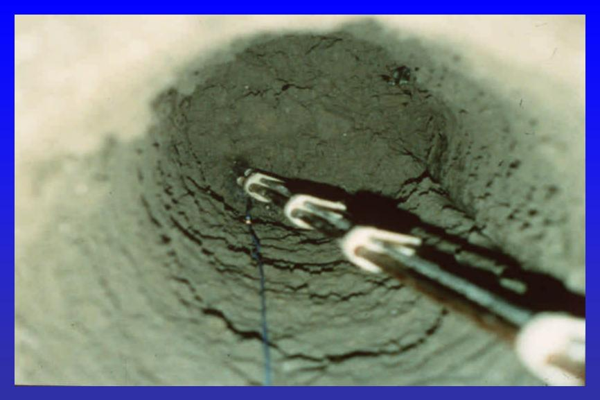
Anode lead wire connection to pipe using spot welder.
