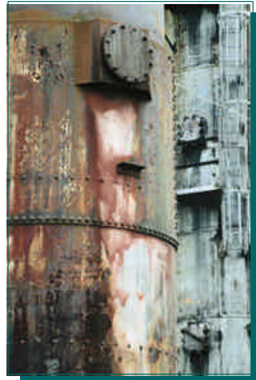
Tanks prior to EcoBond™ preventative coating application
