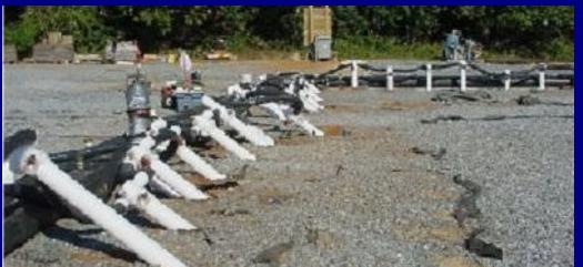
Installed Freeze Pipes (note frost on pipes)
