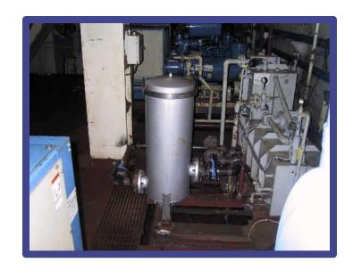
MYCELX filter removing emulsified oil from discharge water on oil drilling ship.
