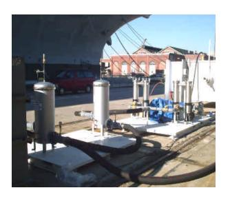
MYCELX filters employed in treatment of Naval bilge water
